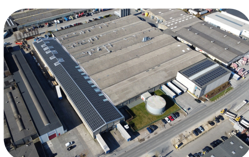
Solar panels - Plastuni Operations
