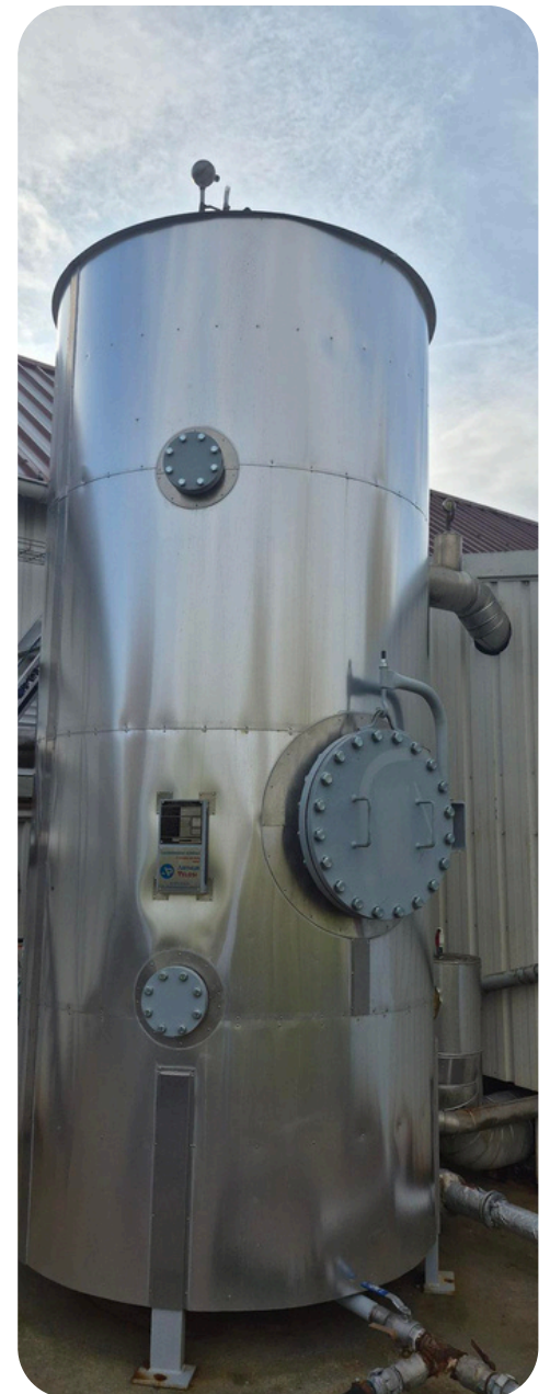
Water tank installed in 2025 Somater Mortagne
