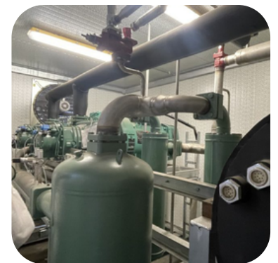
NH 3 refrigeration system - Plastuni Operations
